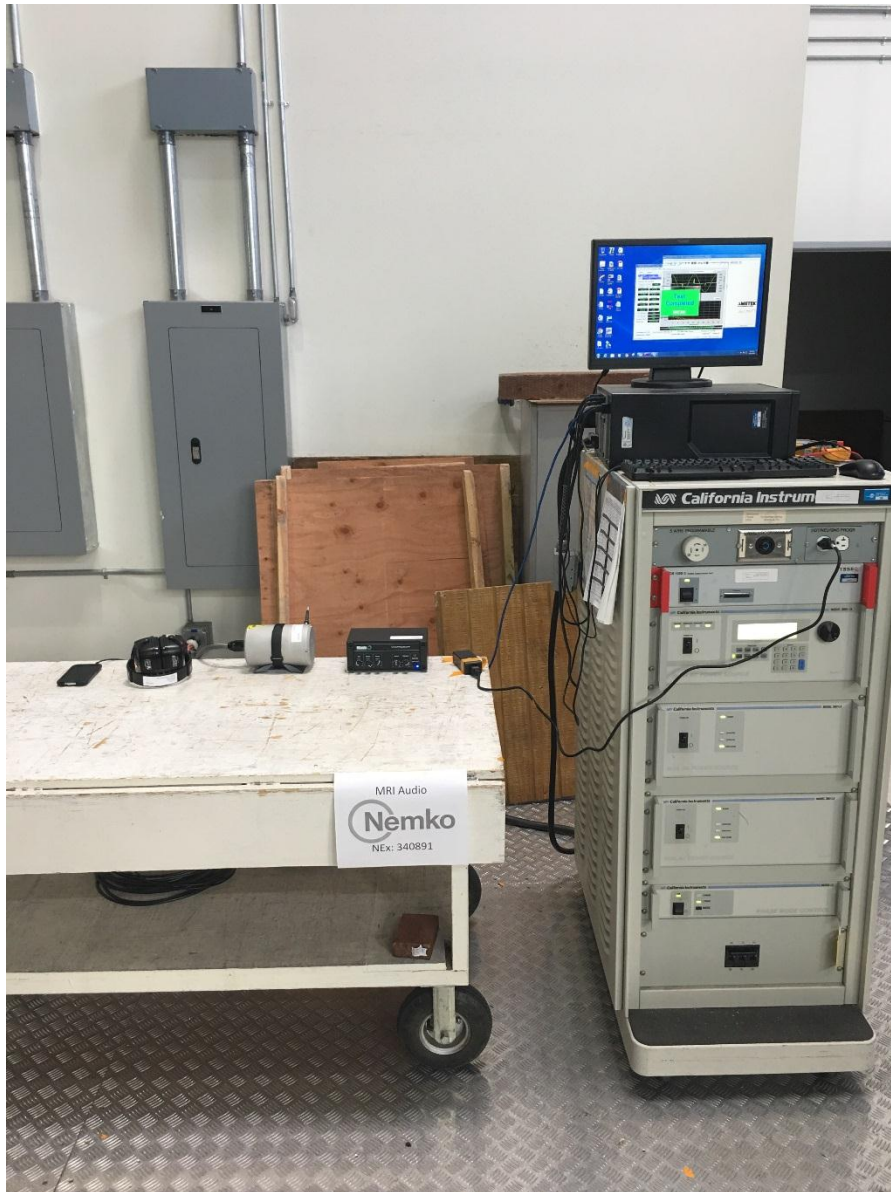
Figure 8.3-1: Harmonic distortion setup photo
